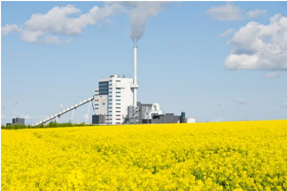
Biofuel-fired CHP-plant in Örtofta
