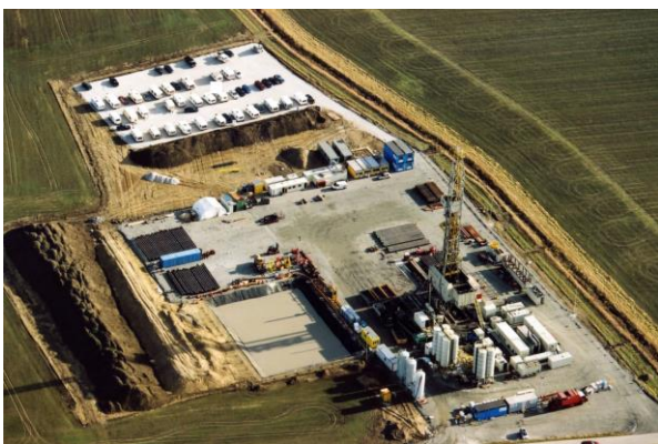
Deep drilling site for a geothermal project. Photo: Perry Nordeng.
